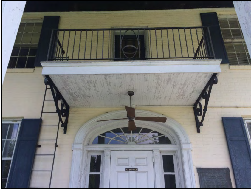
Photograph No. 19: View of the balcony from below.
