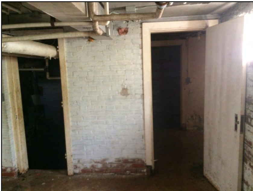
Photograph No. 42: General view of the basement.
