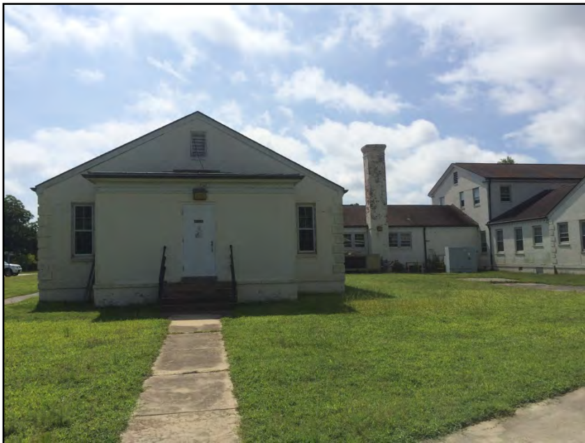
Photograph No. 12: View of the end of the northwest elevation.
