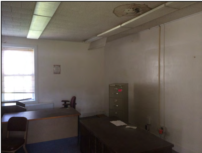
Photograph No. 28: Typical office.
