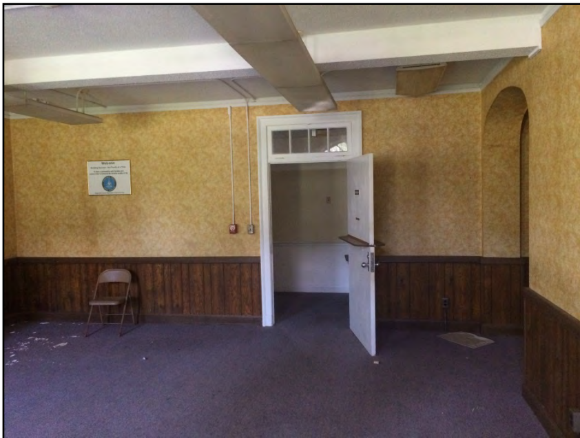
Photograph No. 32: Additional view of the front entrance waiting area.
