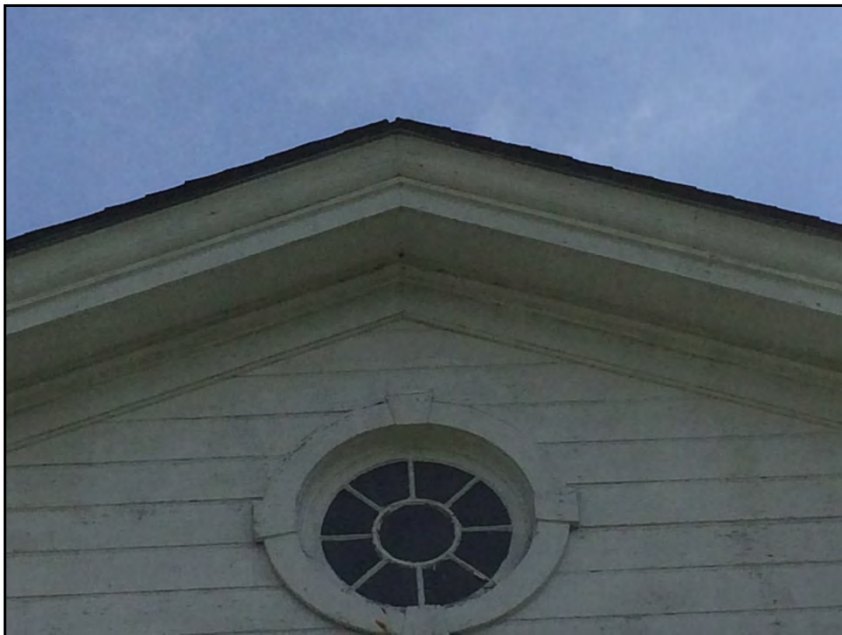
Photograph No. 22: View of the window above the porch.
