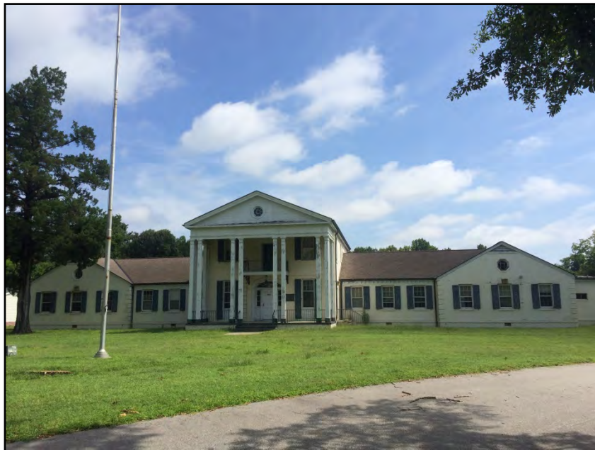
Photograph No. 2: General view of the southwest (front) facing elevation.
