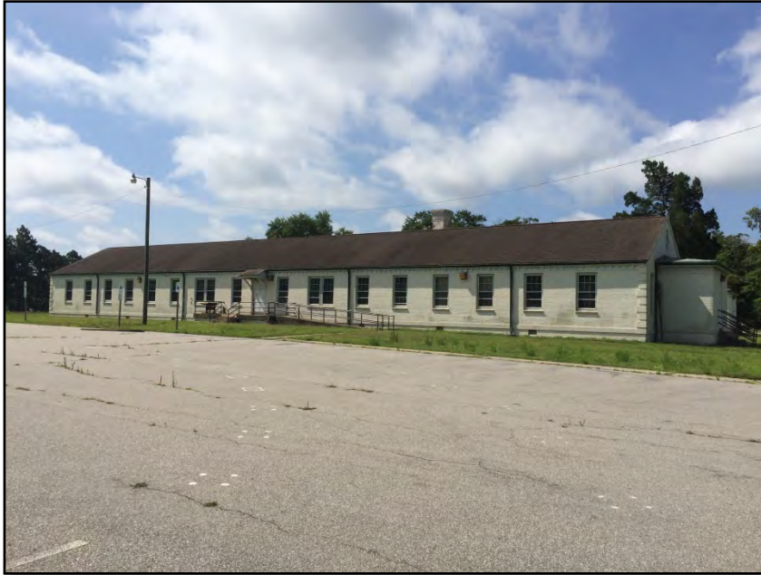
Photograph No. 11: View of the north facing (rear) elevation.
