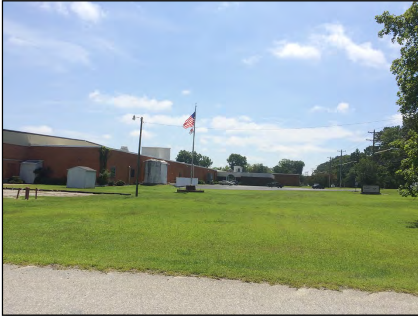
Photograph No. 59: View of Glenoit Fabrics looking east toward the Subject Property.
