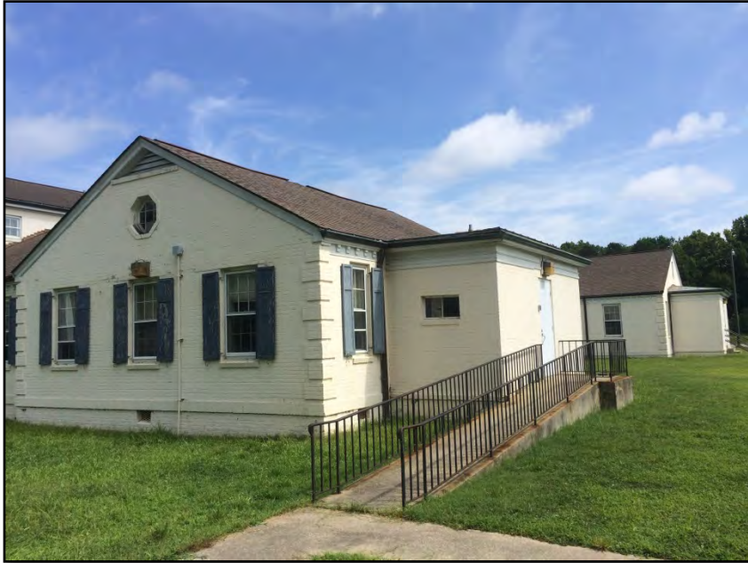
Photograph No. 5: View of the east end of the southeast wing.
