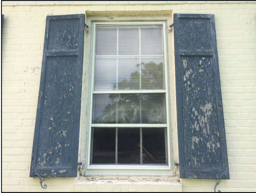
Photograph No. 23: Typical window.
