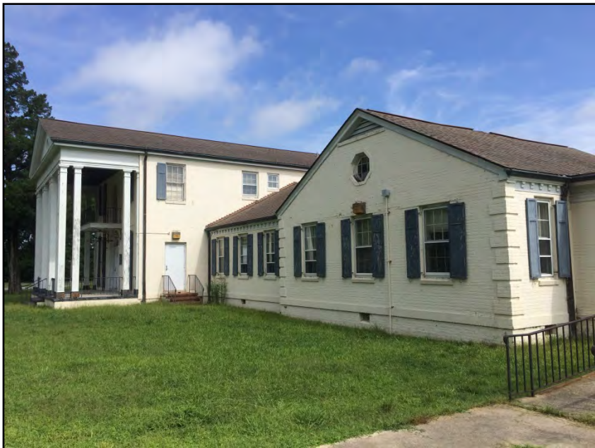
Photograph No. 4: View of the southeast wing.
