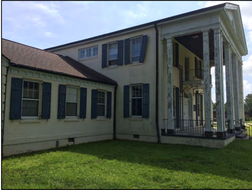
Photograph No. 17: Additional view of the front porch.
