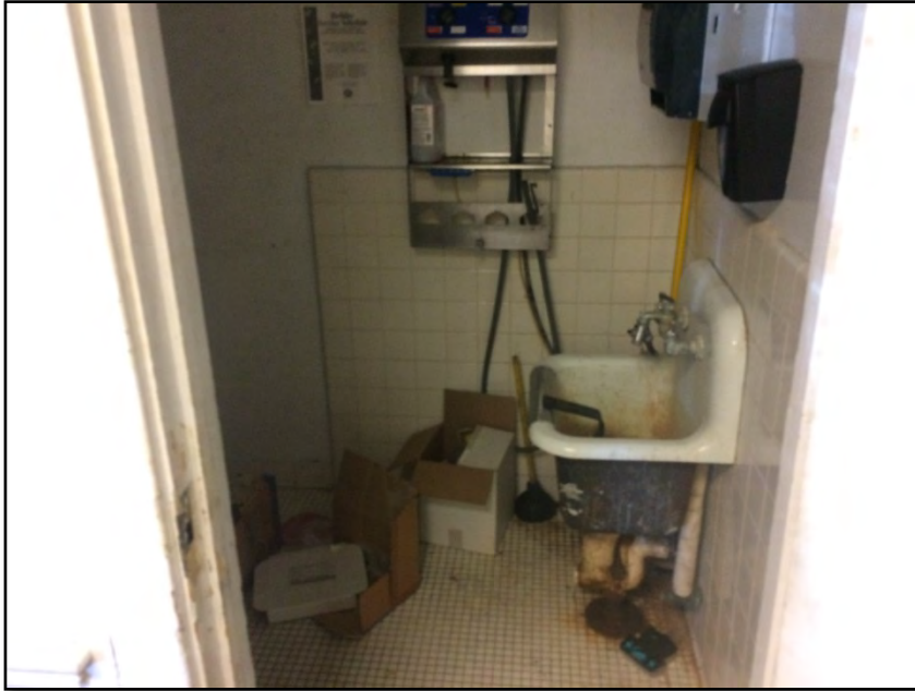
Photograph No. 37: View of a utility closet.
