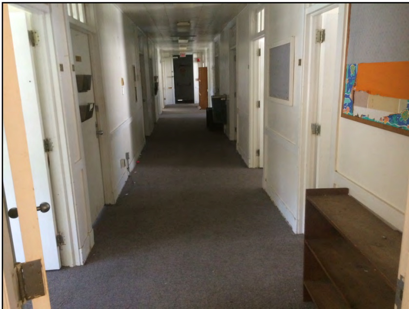
Photograph No. 26: Typical view of the interior hallways.
