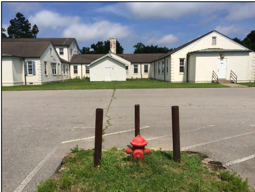
Photograph No. 6: General view of the east facing elevation.
