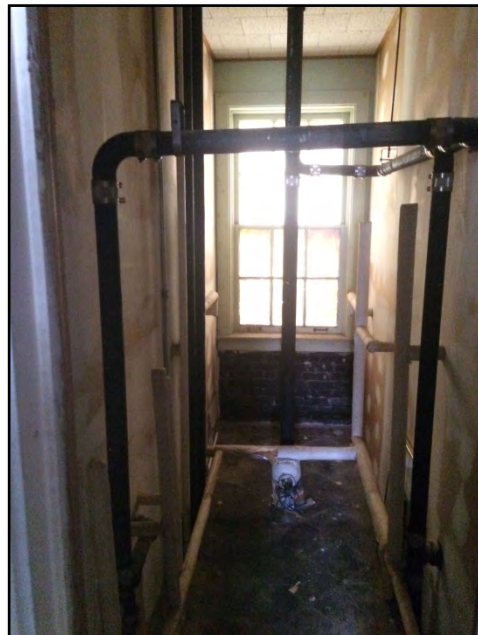
Photograph No. 40: View of a pipe chase closet.
