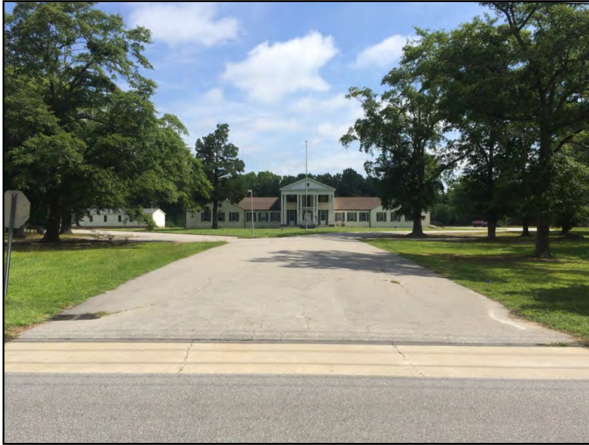
Photograph No. 47: View looking northeast toward the building.
