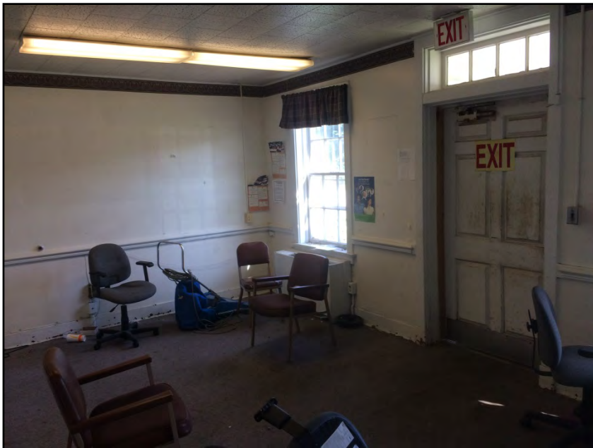
Photograph No. 24: View of the rear entrance located between the northwest and northeast wings.
