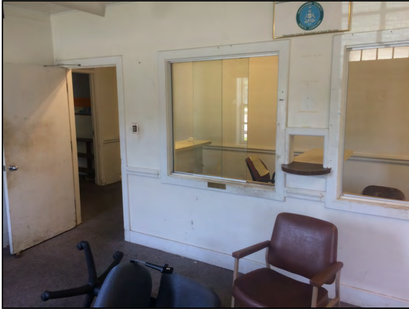
Photograph No. 25: View of the rear office.
