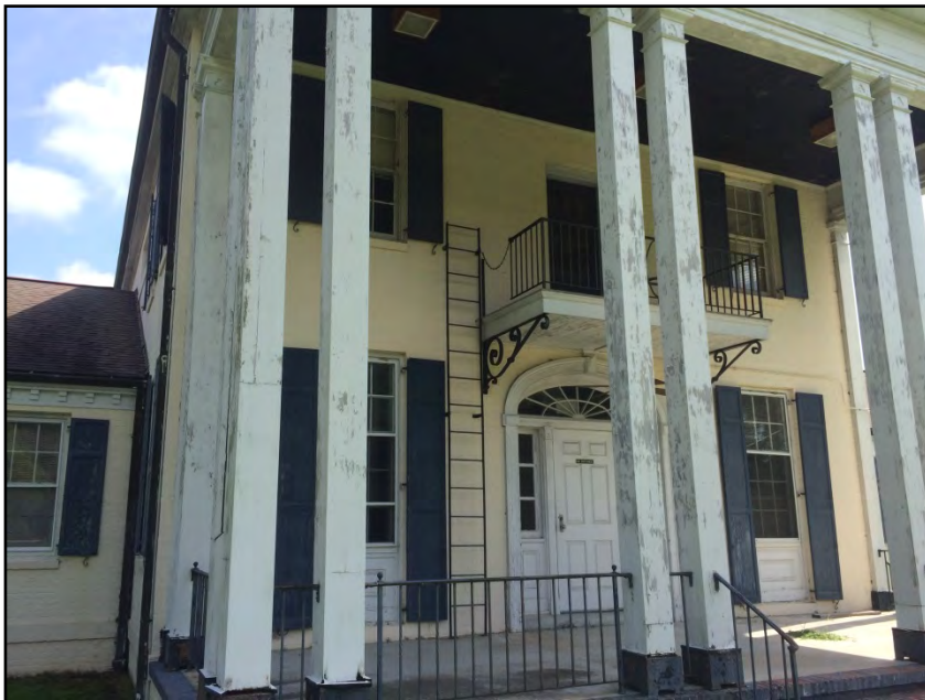
Photograph No. 18: Additional view of the front porch.
